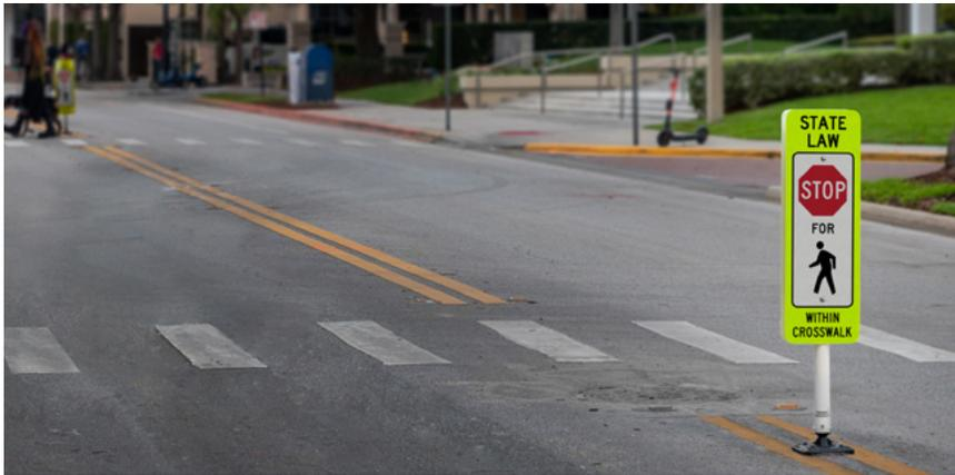
The In-Roadway Pedestrian Crossing sign is designed to be placed on the centerline in advance of a midblock crosswalk to remind drivers they are required to stop for pedestrians who are waiting to cross or are crossing.
